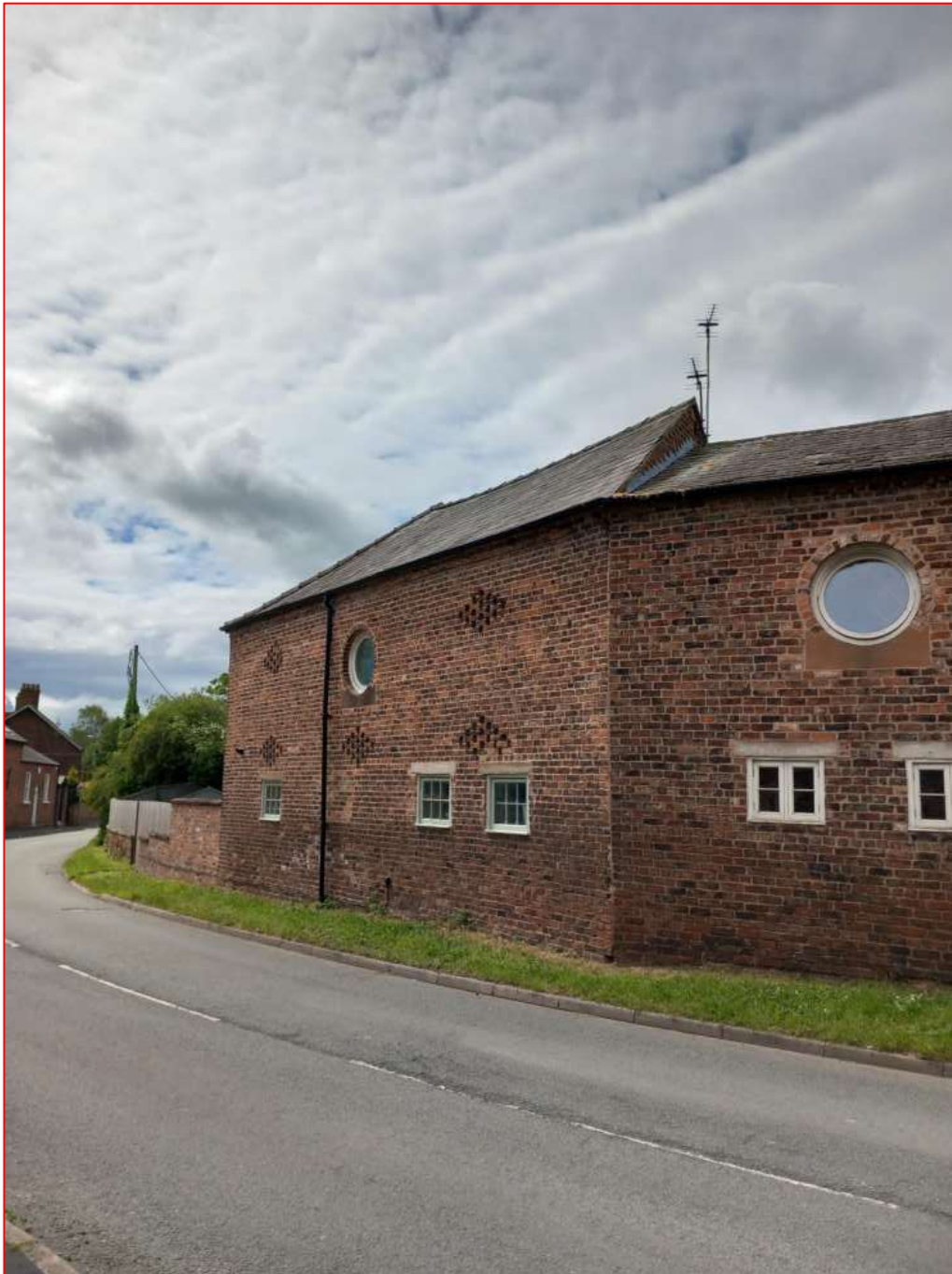
Plate 22: Farm buildings at Laurel Farm (NHLE: 1320457)
