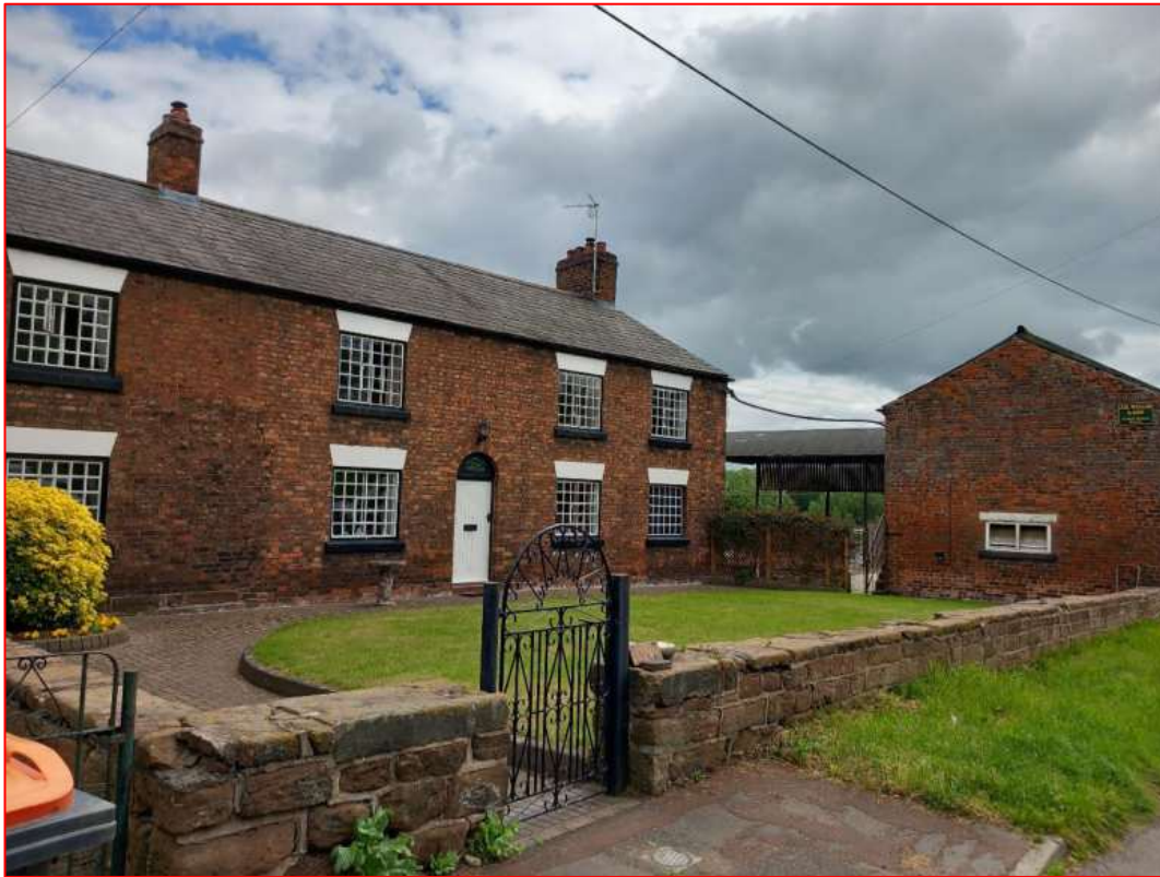
Plate 12: Lower Green Farmhouse with wall to front garden (NHLE: 1086967)
