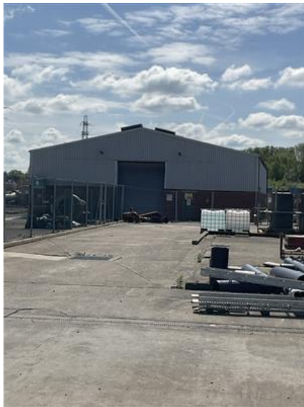
Photograph 43 – Brick and metal sheet cladding building
