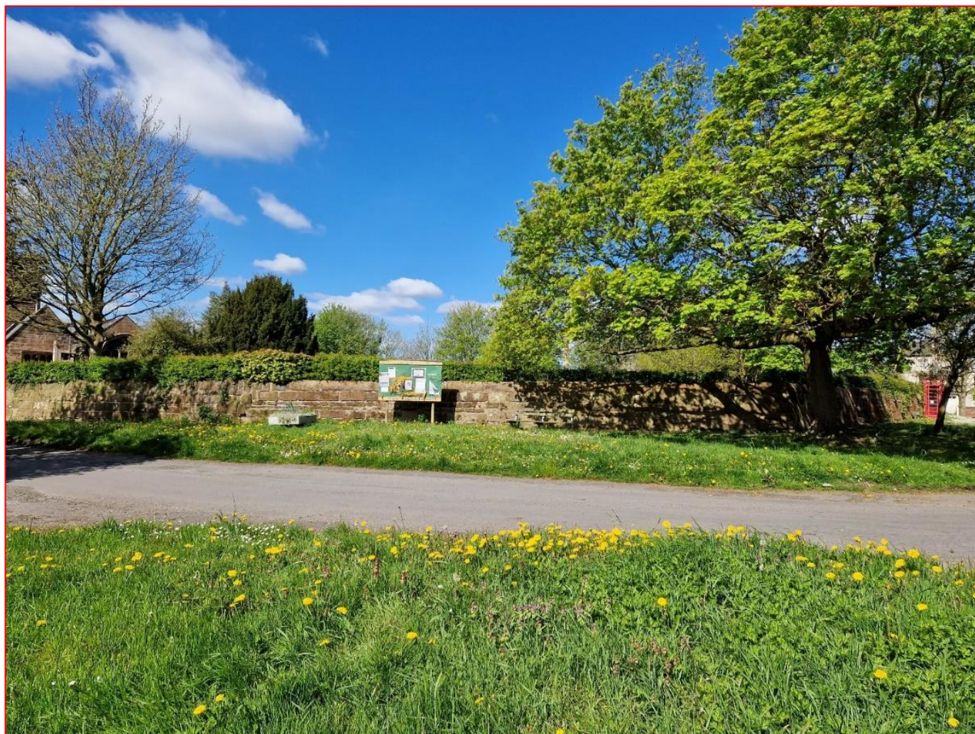
Plate 42: View of the southern and eastern retaining walls of the Church of St Mary, facing northwest
