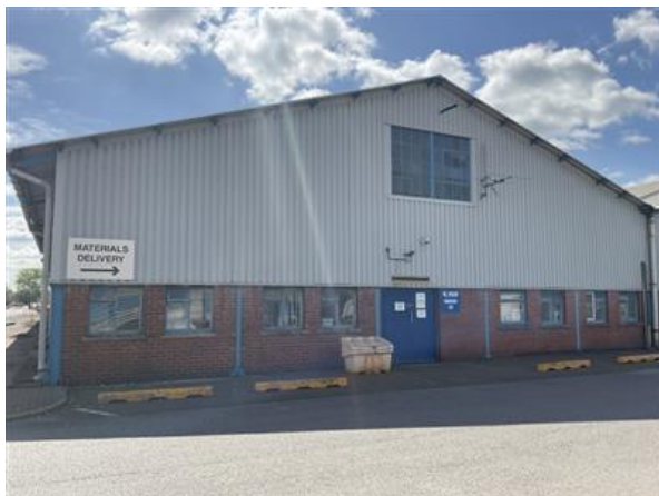
Photograph 45 – Brick and metal warehouse
