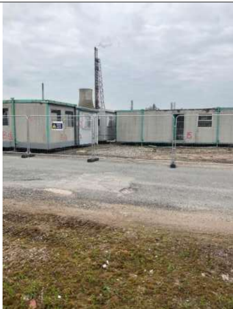
TN1 – Active demolition site
