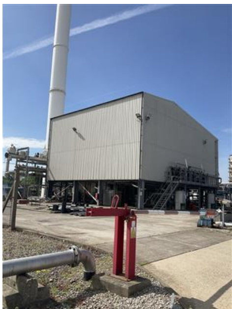
Photograph 41 – Metal clad building
