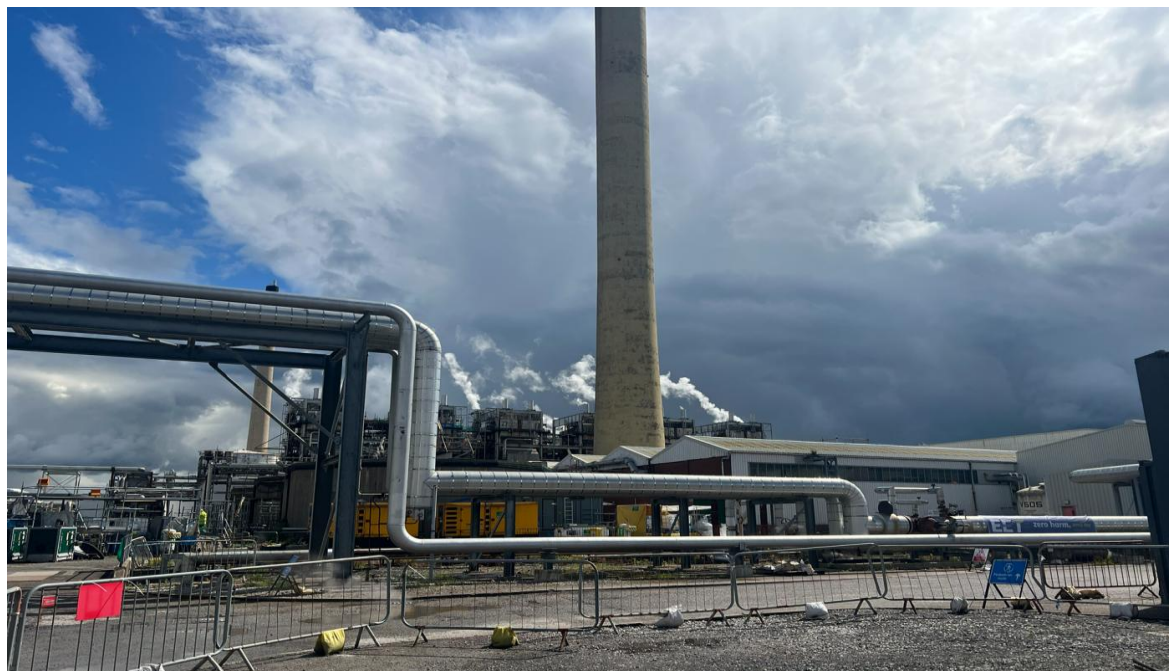
Photo 4: Infrastructure on site
