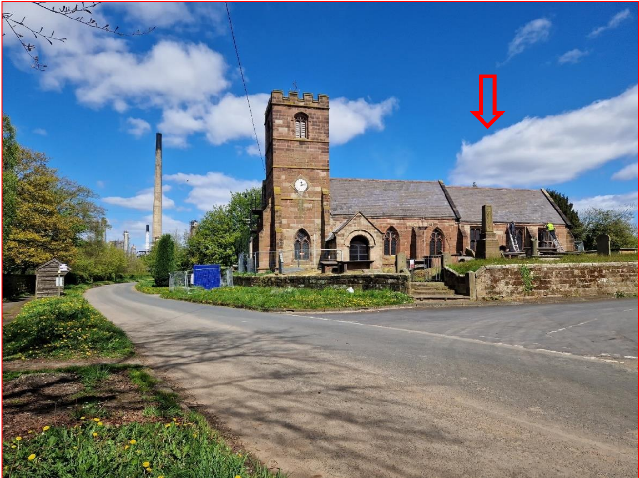
Plate 38: View of the Church of St Mary looking towards the SMC, facing north. The War Memorial (arrowed) is visible within the graveyard, with the retaining walls enclosing the Church grounds
