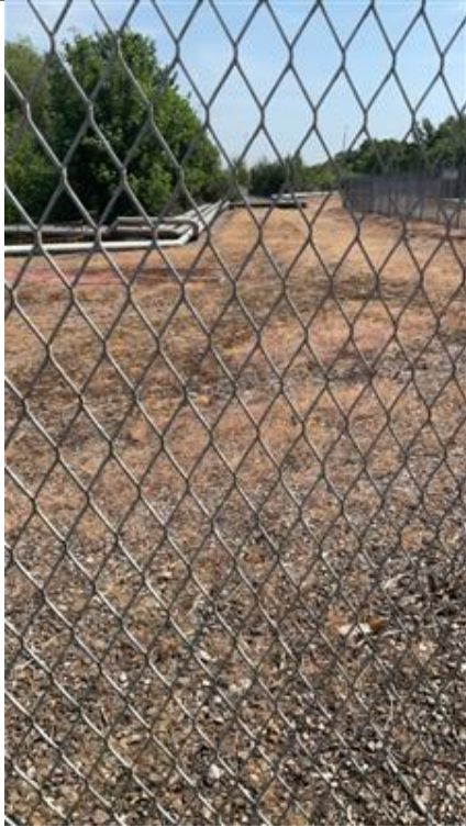
Photograph 51 – Unsealed ground to the north of Oil Sites Road
