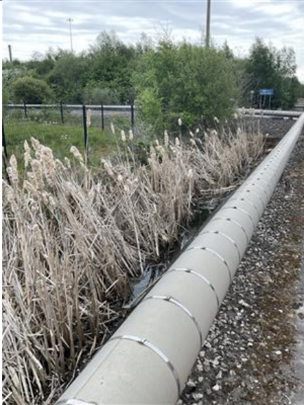
Photograph 59 – Concrete-banked draining ditch
