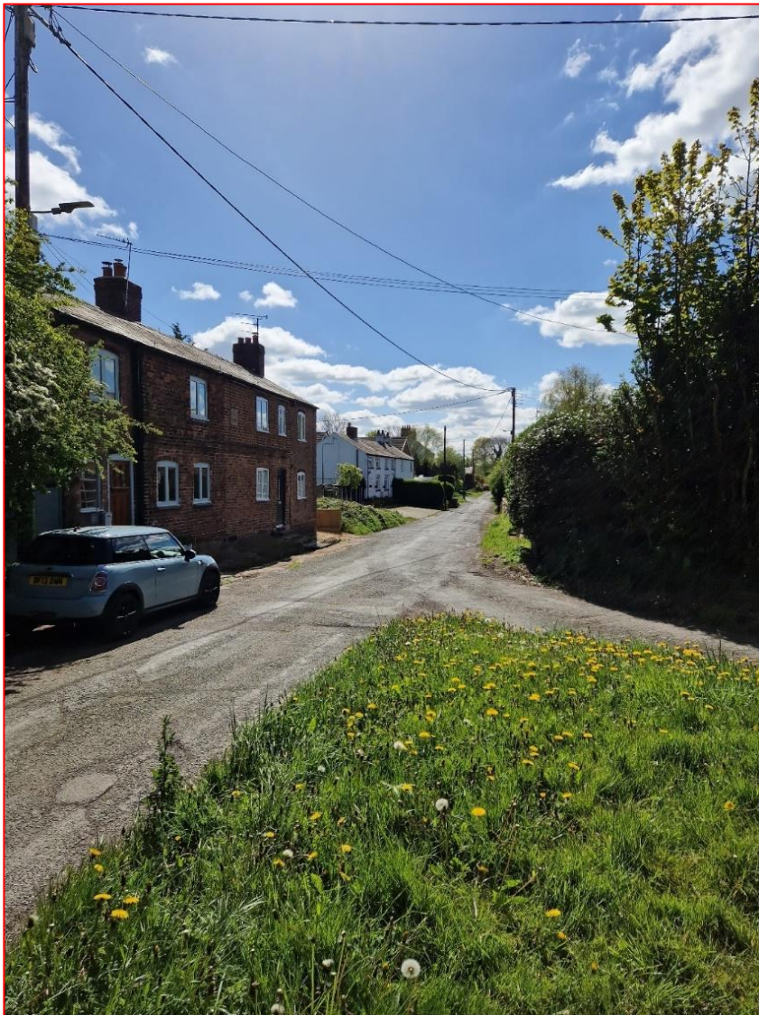
Plate 33: View from the junction of Poole Lane and Thornton Green Lane, facing southeast towards the southern part of the Conservation Area
