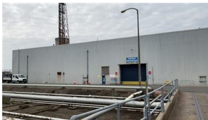
Photograph 38 – Metal corrugated building
